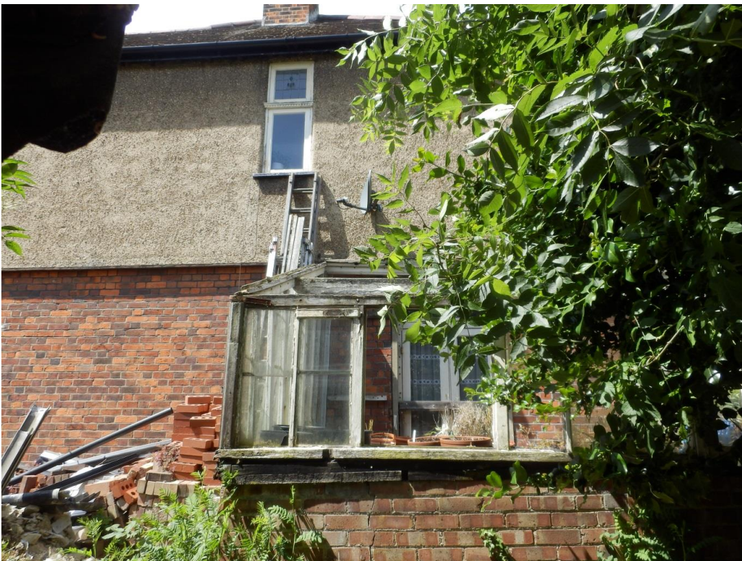
Conservatory in use as plant nursery
