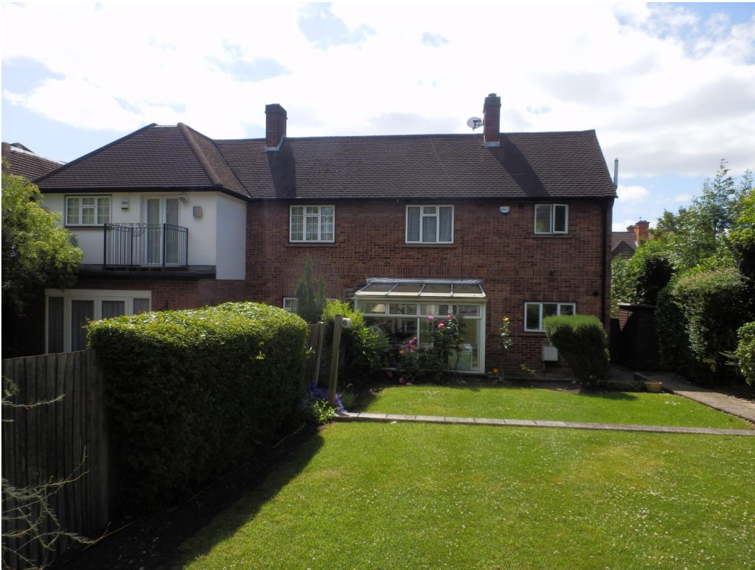
Rear elevation, with no. 14 to the left; no. 14's existing two-storey extension visible
